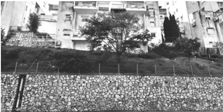
Retaining walls as a functional necessity: Retaining wall on Hazan Street in Haifa, Photo: Original, 2025
