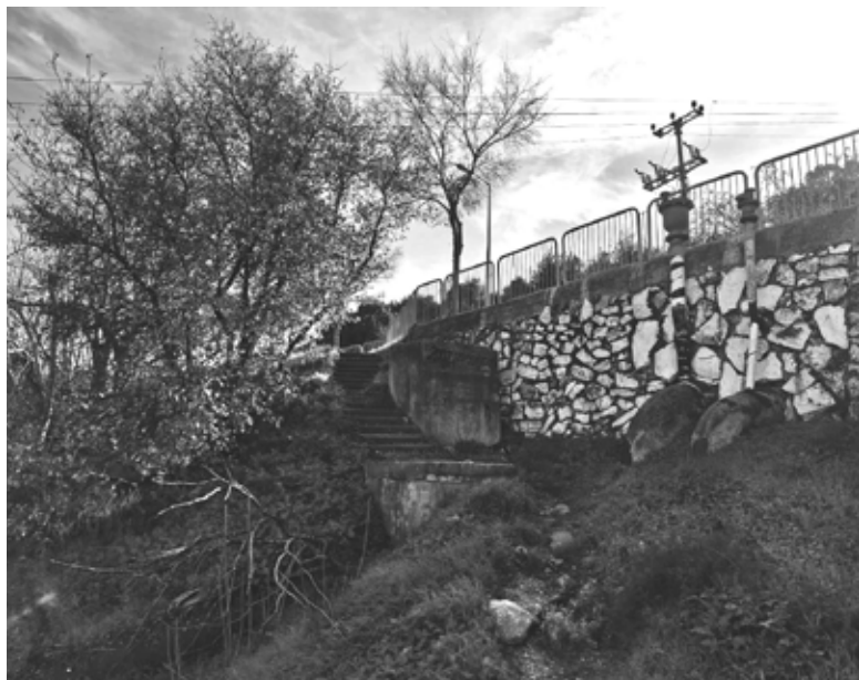
Open space potential: improvised paths in an overlooked area. Photo: Original, 2025
