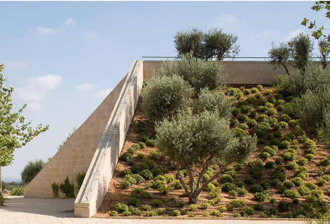
,Between Architecture and Landscape: Yad Hanadiv Visitors Center, Ramat Hanadiv Arch. Ada Carmi-Melamed, Photo: Amit Guron, 2008
